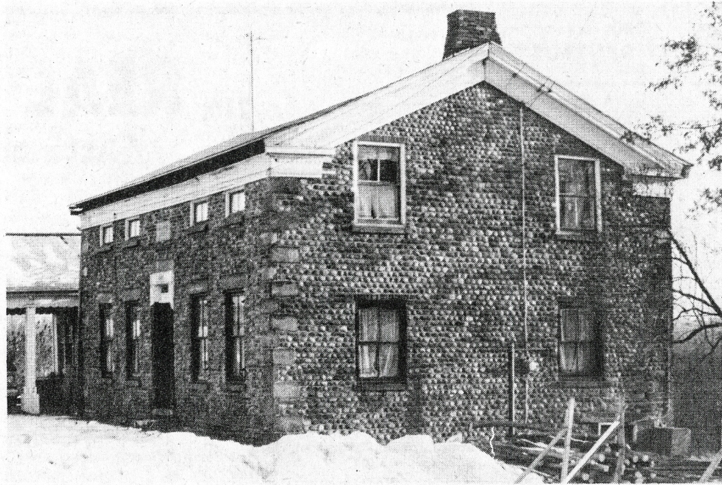
MACOMBER HOUSE--Photo shows cobblestone on Ridge in Murray, taken in 1975, before canopy was removed.
